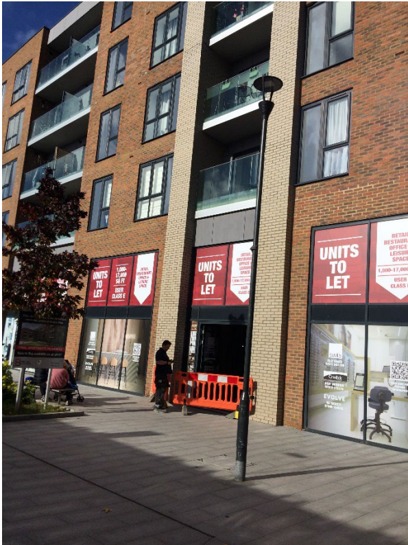
View of Premises Entrance
